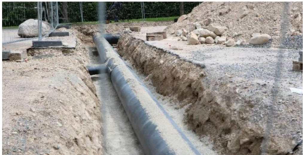
Figure 21: Alabastern: biomass-based low-temp DH-supply.
