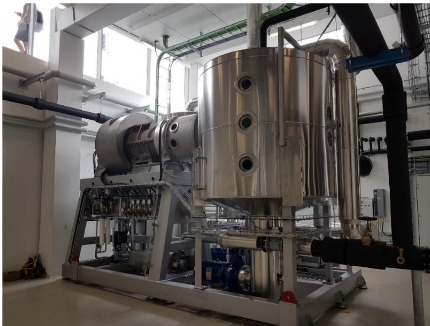
Figure 10: New type seawater heat pump with water as refrigerant
