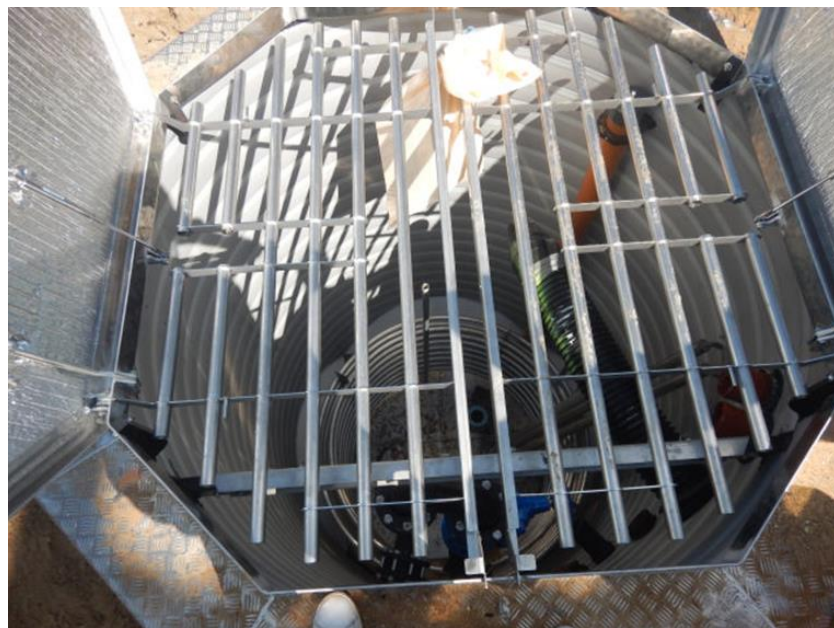
Figure 11: Manhole and installed heat exchanger of the wastewater heat recovery system in Aarhus (DK2)
