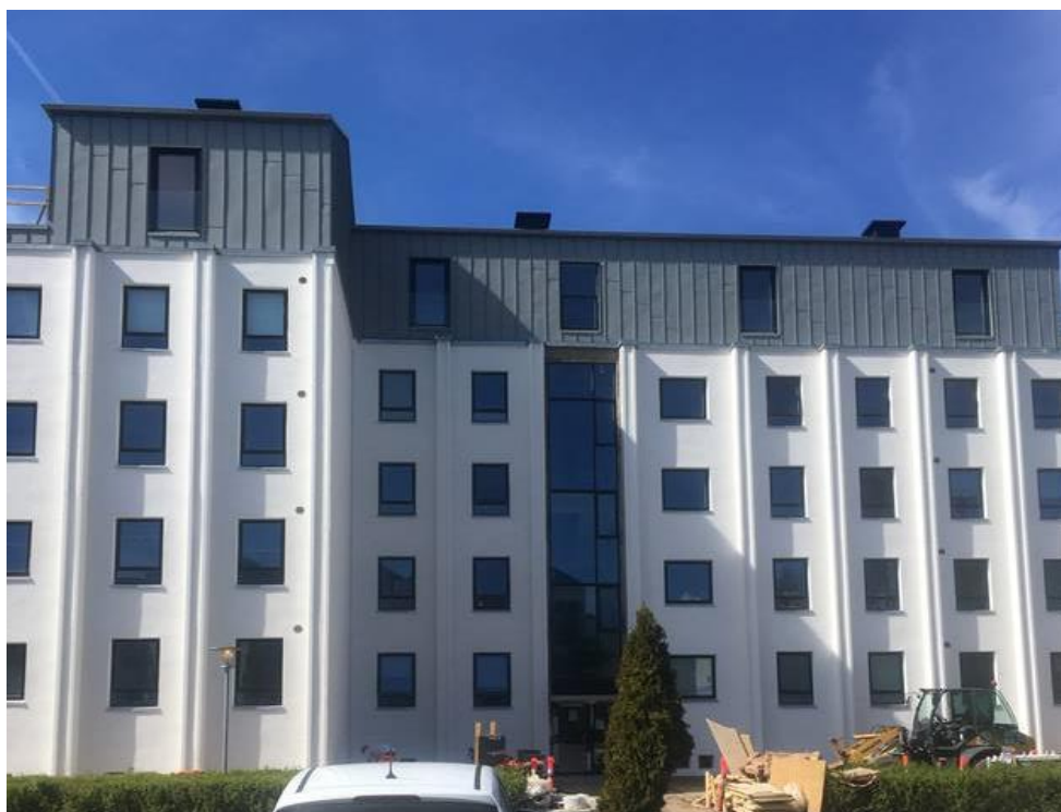
Figure 10. Buildings in District 21 Rydevænget/Fjældevenget, Aarhus (RDS DK1) after refurbishment 13
