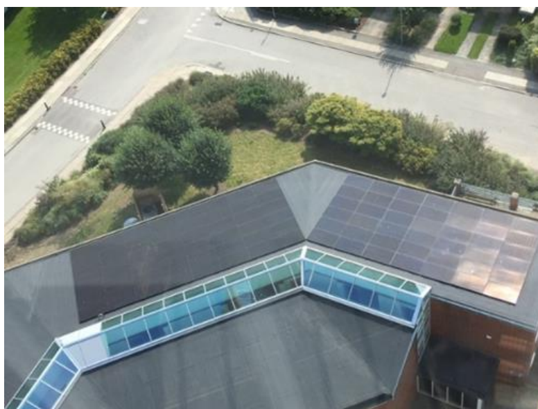
Figure 25: View of the installed PV system on the office building's roof in Dybedalen 1A (RDS DK3)
