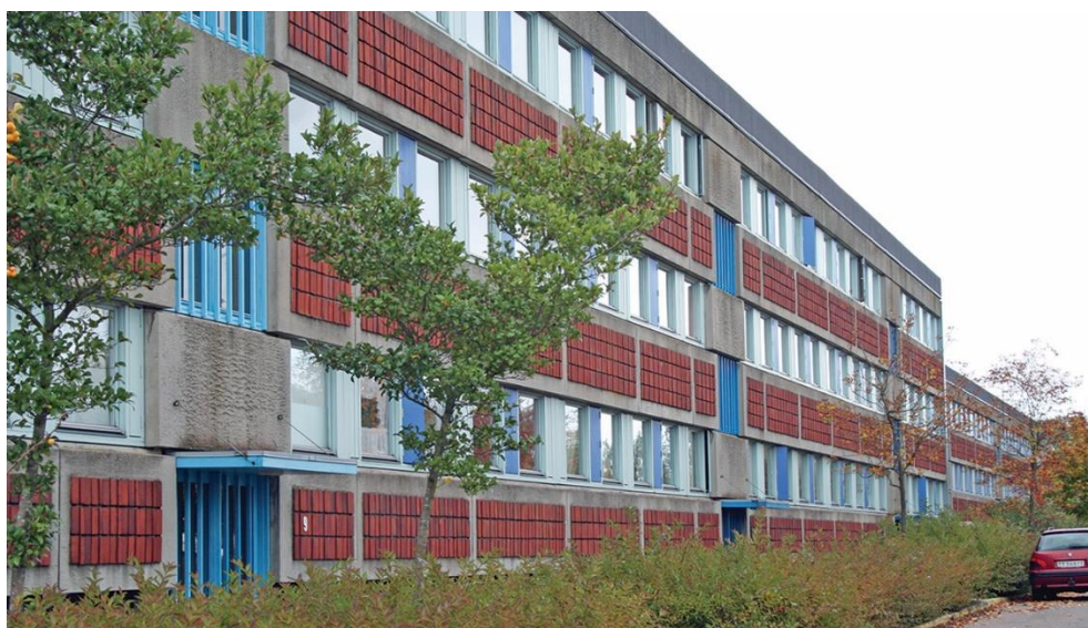
Figure 11: Buildings in District 20 Trigeparken, Aarhus (RDS DK2) before refurbishment
