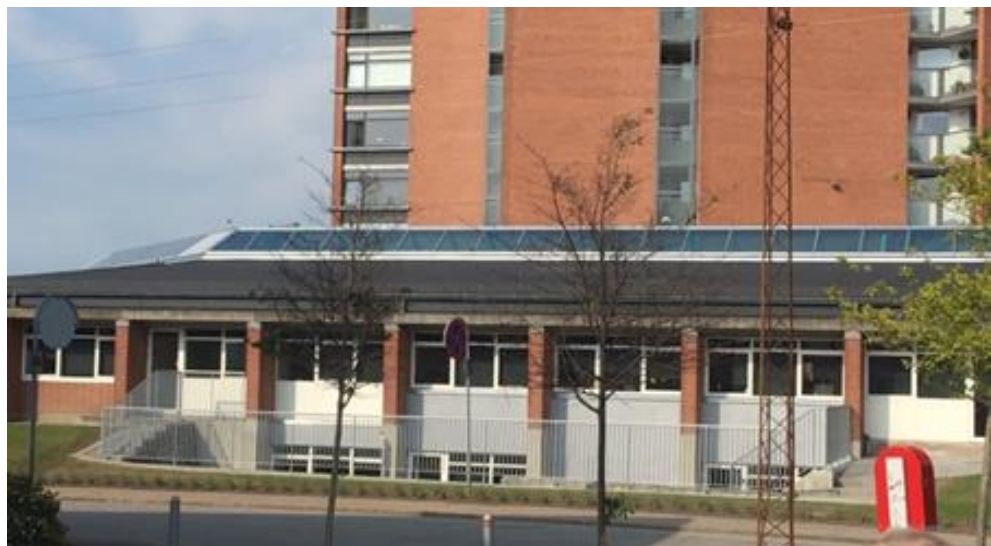
Figure 13: Office building located in Dybedalen 1A (RDS DK3)
