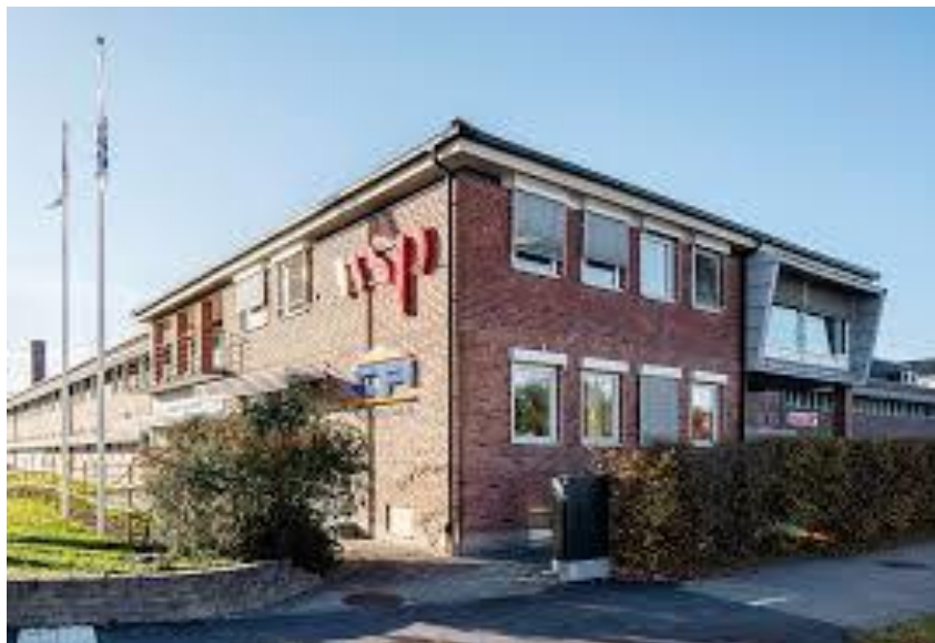
Figure 17: Monitored office building located in Tvinnaren 4 (RDS SE3) 17
