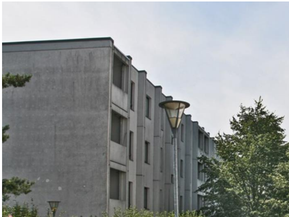
Figure 9: Buildings in District 21 Rydevænget/Fjældevænget, Aarhus (RDS DK1) before refurbishment 12
