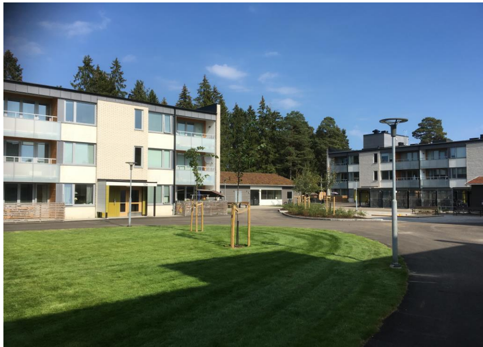
Figure 15. Monitored buildings in Alabastern, Växjö (RDS SE1) after refurbishment
