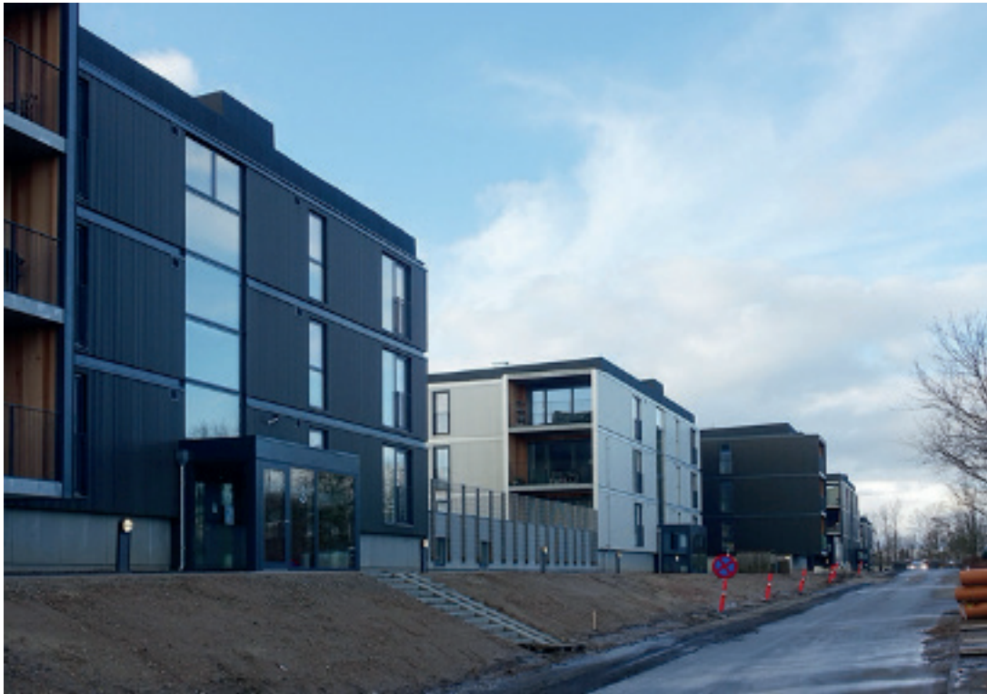
Photo: READY demonstration site for near Zero-Energy Buildings and Smart Energy Systems in Trigeparken, Aarhus Denmark.
