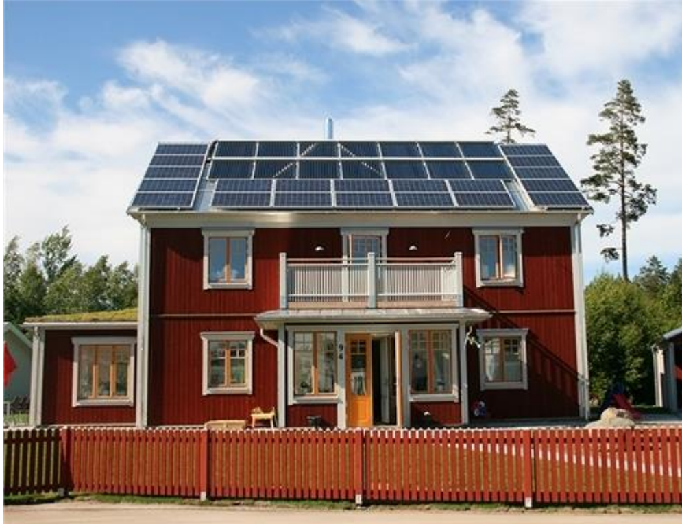
Picture 14 – Åsaliden, Växjö - An energy plus house with heat driven appliances [14]
